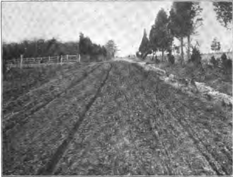
1 Columbus and Burlington road, Burlington Co., before improvement.
